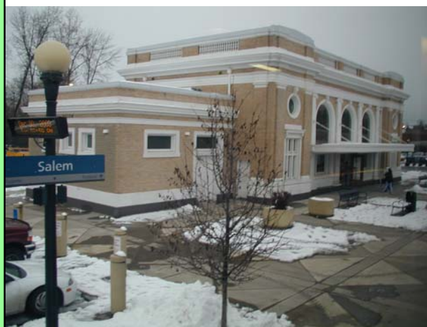
The refurbished Salem, Oregon station.
