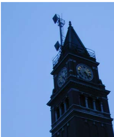
The King Street Station clock tower.
