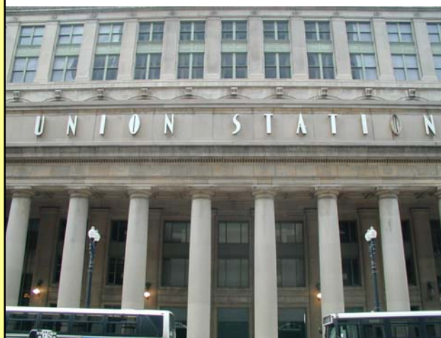
The main entrance to Union Station.
