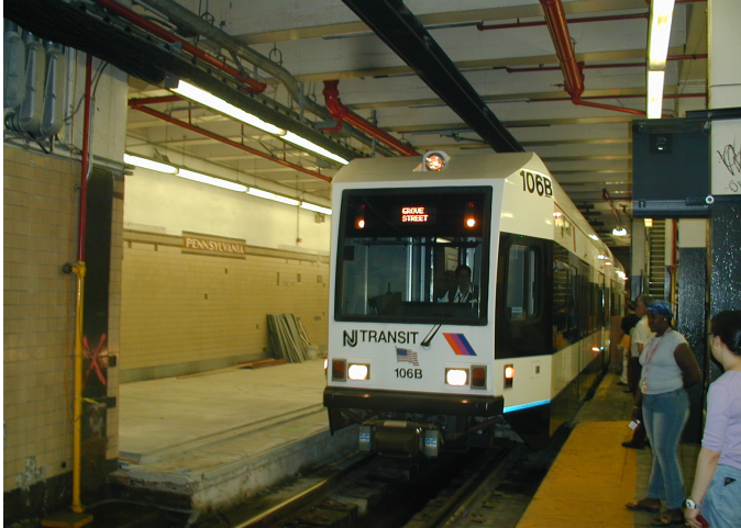
A NJT light-rail arrives at the Newark City Subway Station under Newark Penn Station.
